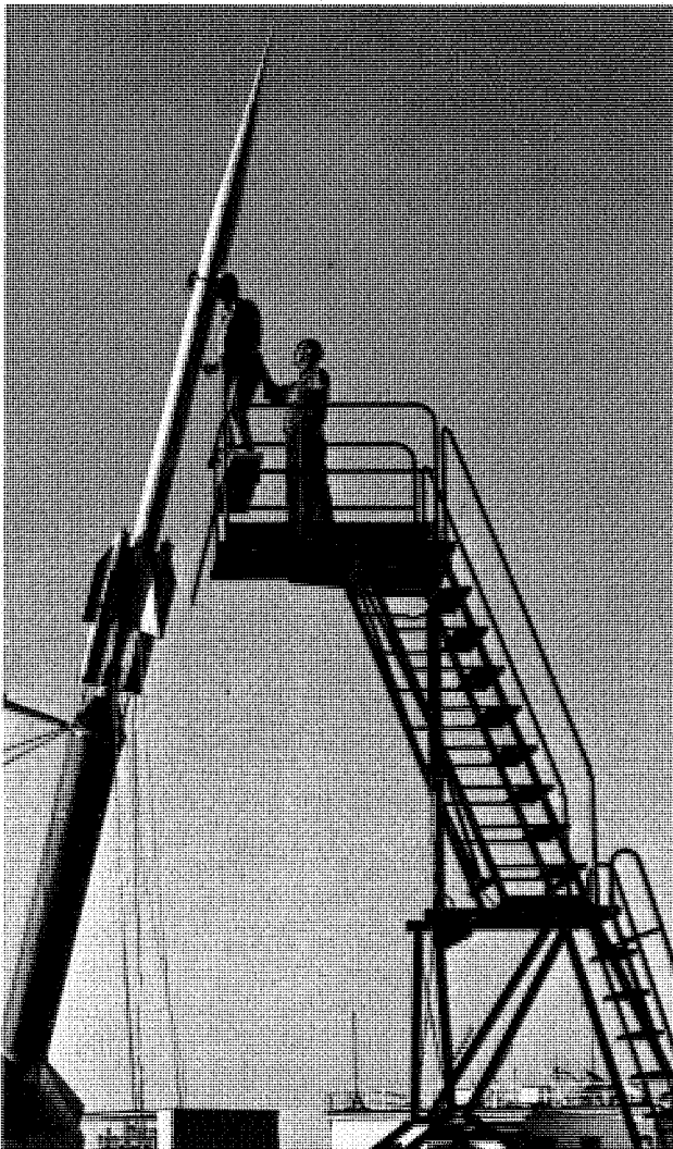
FIGURE 255. Technician Roy Hindle makes an adjustment to F23 roll-stabilized ramjet model as E. R. Matthews lends a supporting hand in preparation for Wallops launch of the model with a Nike booster, September 24, 1954.
