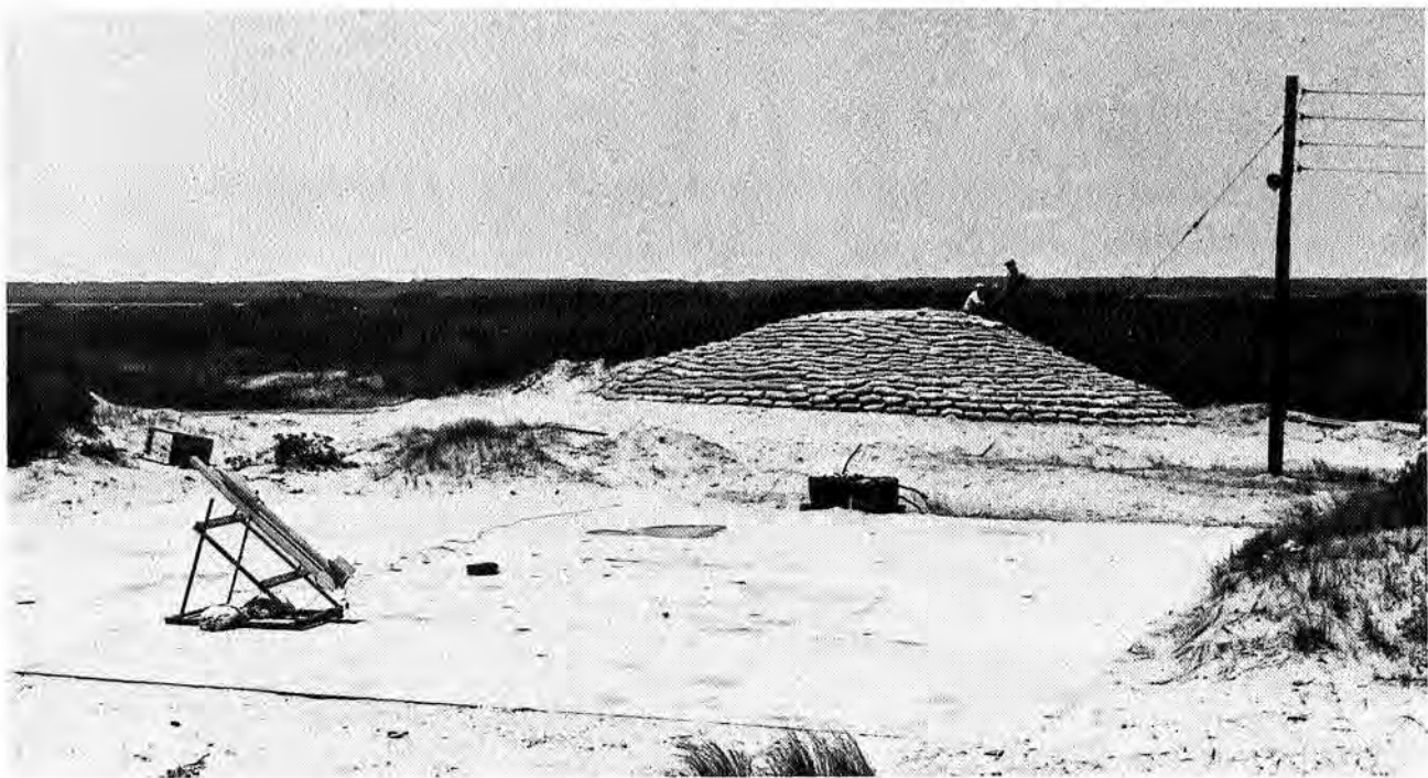
FIGURE 23. Wallops launch slab and blockhouse, June 1945.
