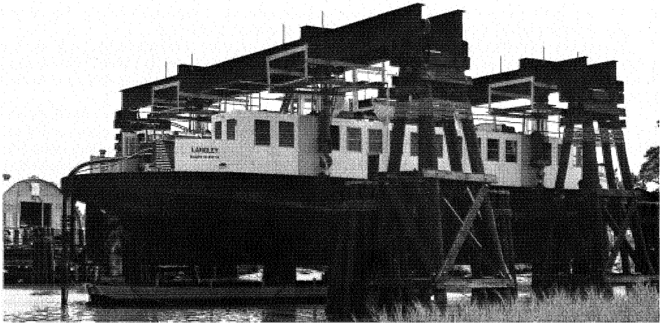
FIGURE 151. The Ferry Langley shown in raised position as it undergoes bottom maintenance in ferry slip at Mainland Dock, July 13, 1954.
