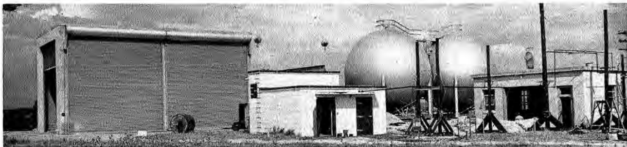
FIGURE 73. Exterior view of Wallops Island Preflight Jet test unit.
