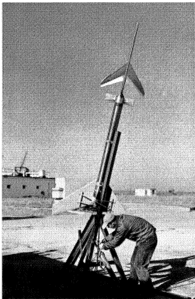
FIGURE 206. Technician George Cutler checks launcher for one of the E34 series of wing-drag research models, December 17, 1952.
