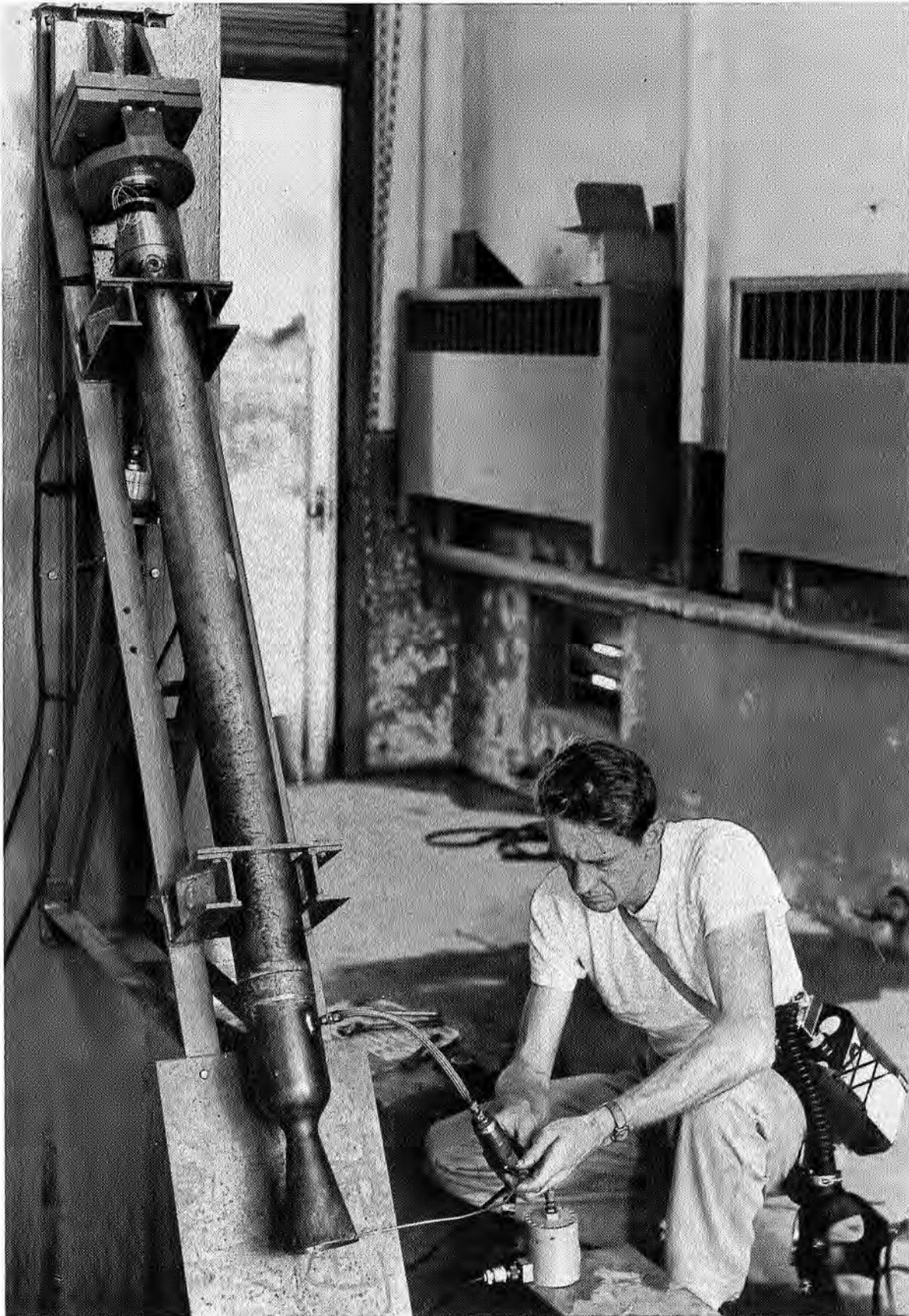
FIGURE 89. Propulsion technician Carl G. Baab readies British Typhoon liquid-rocket motor for firing. Rocket is shown in Wallops rocket test cell, June 6, 1951.
