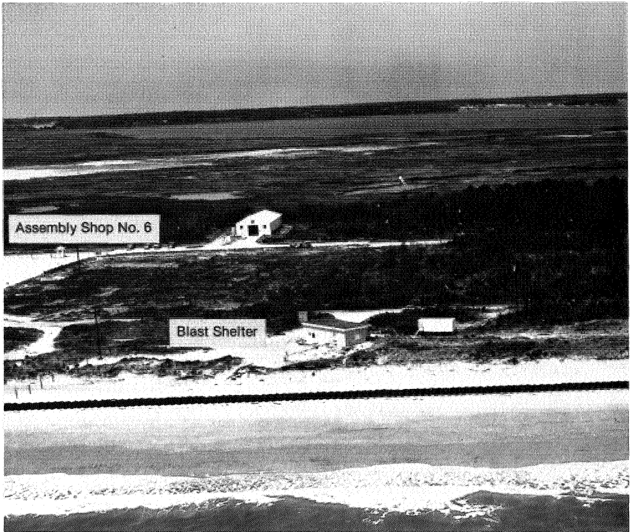
FIGURE 280. Aerial view of north area of Wallops Island showing blast shelter and Assembly Shop No. 6.
