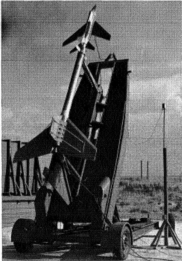
FIGURE 218. Rocket model of North American YF-100A airplane with Deacon booster, shown at Wallops, November 7, 1952.
