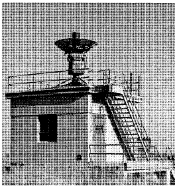
FIGURE 247. Fiberglass enclosure over Rawinsonde antenna at Camera Station 2. Wallops, February 14, 1955.
