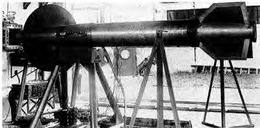
FIGURE 74. Lewis 16-inch ramjet flight test unit in 12-inch nozzle of Wallops Preflight Jet.
