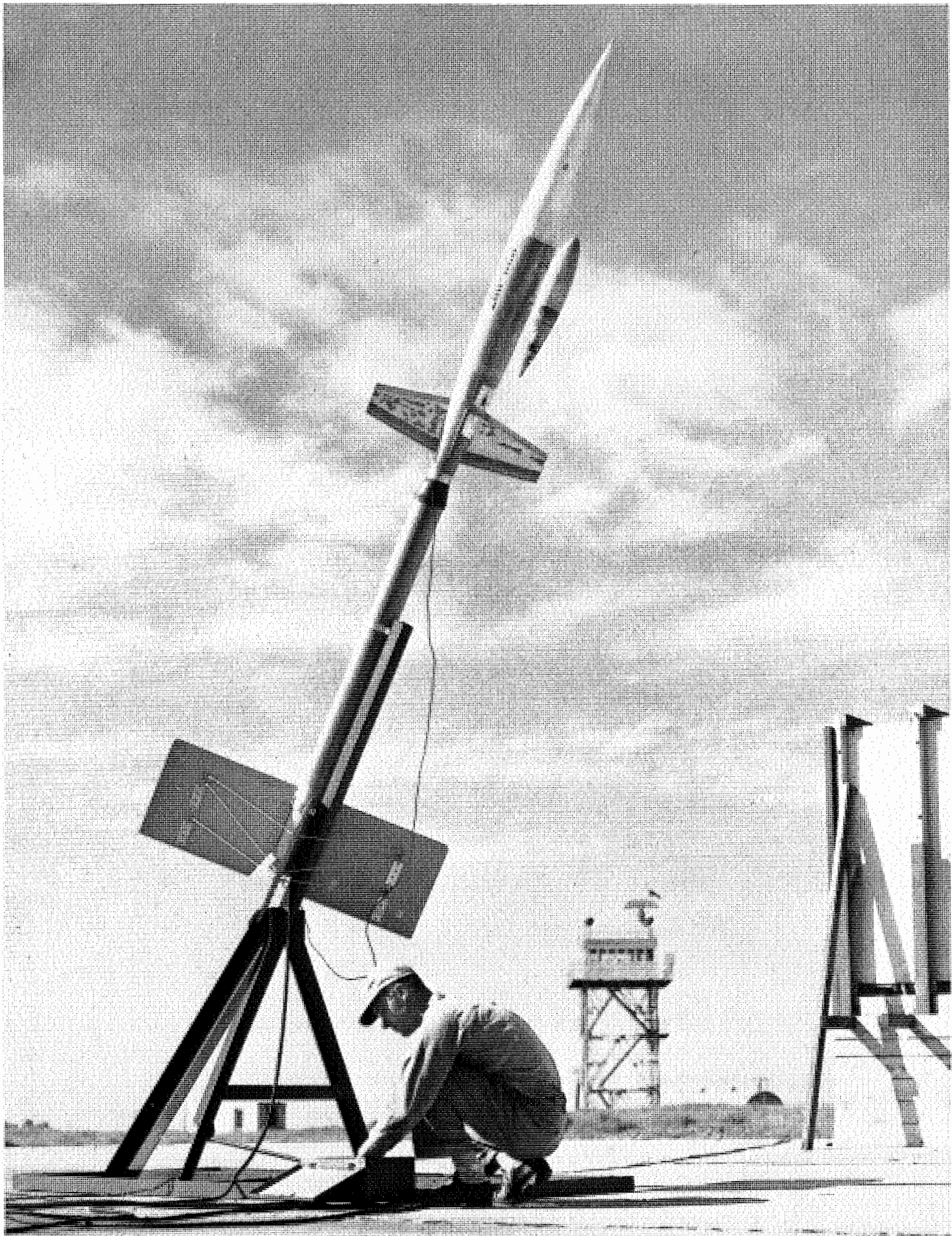
FIGURE 172. Technician Durwood Dereng checks the firing leads of HPAG booster for D28 buffeting-research model with a large external store, May 6, 1952.
