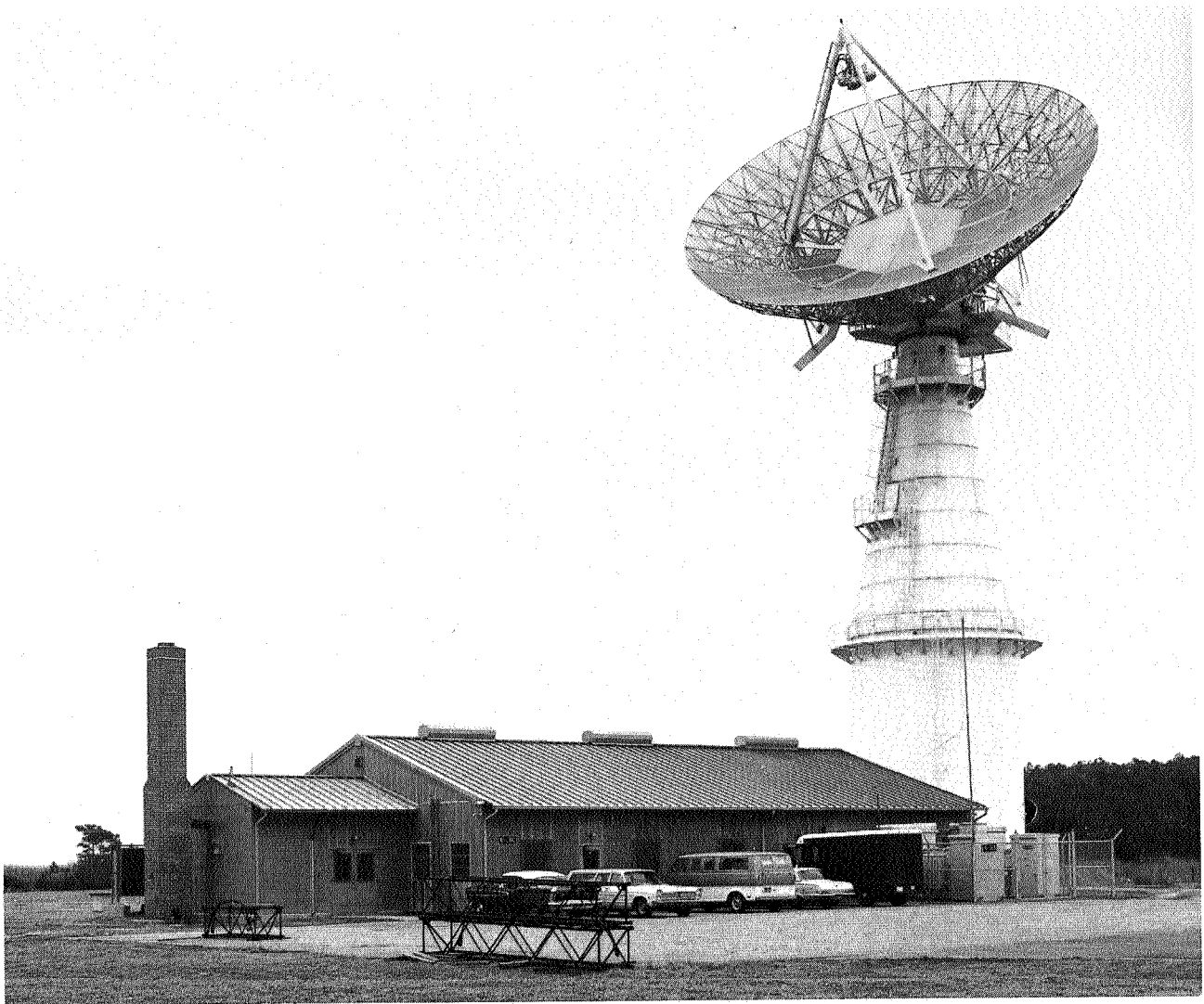
FIGURE 418. View of Spandax radar on mainland near Wallops Island.
