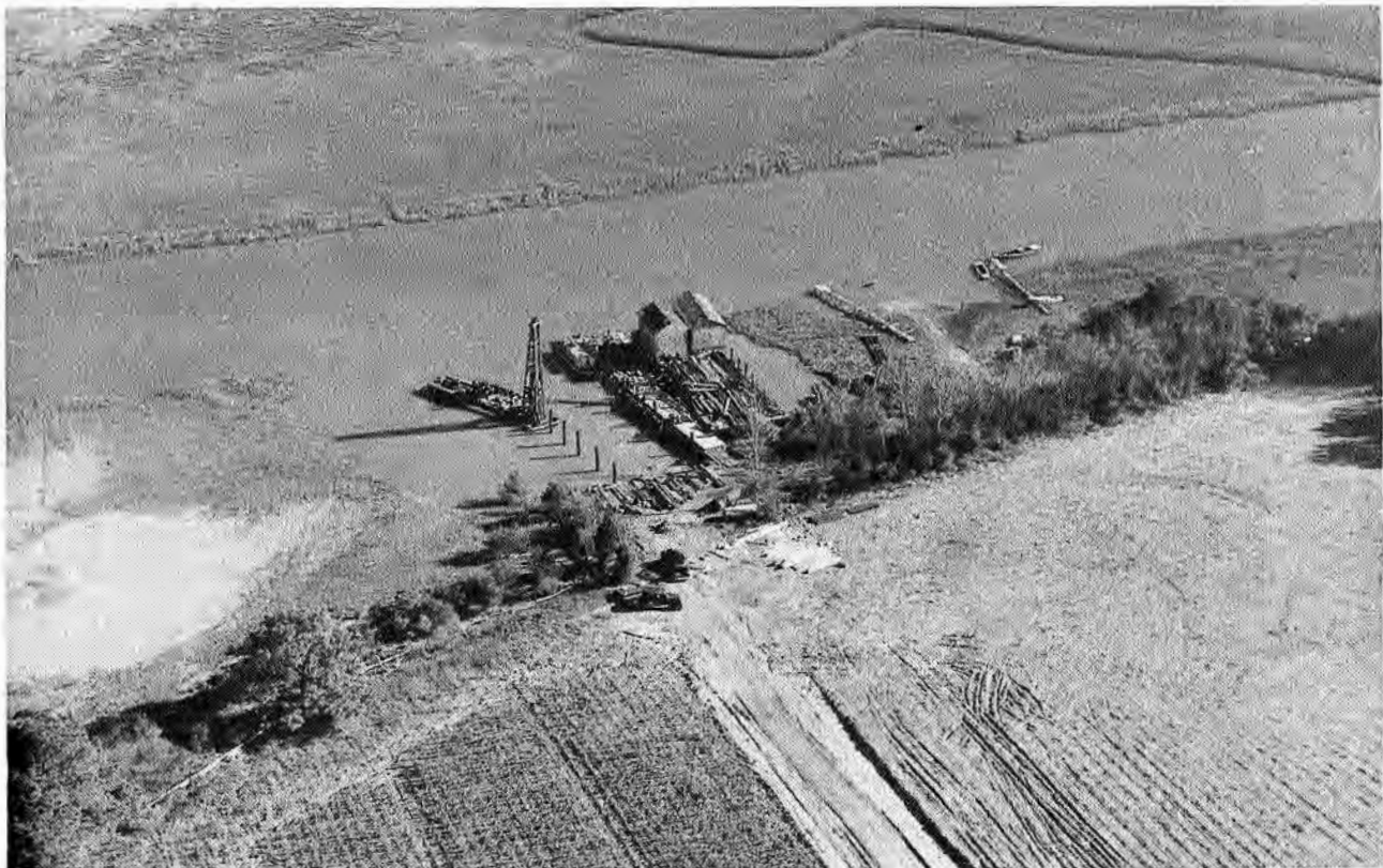
FIGURE 17: Mainland Dock under construction, January 1946.
