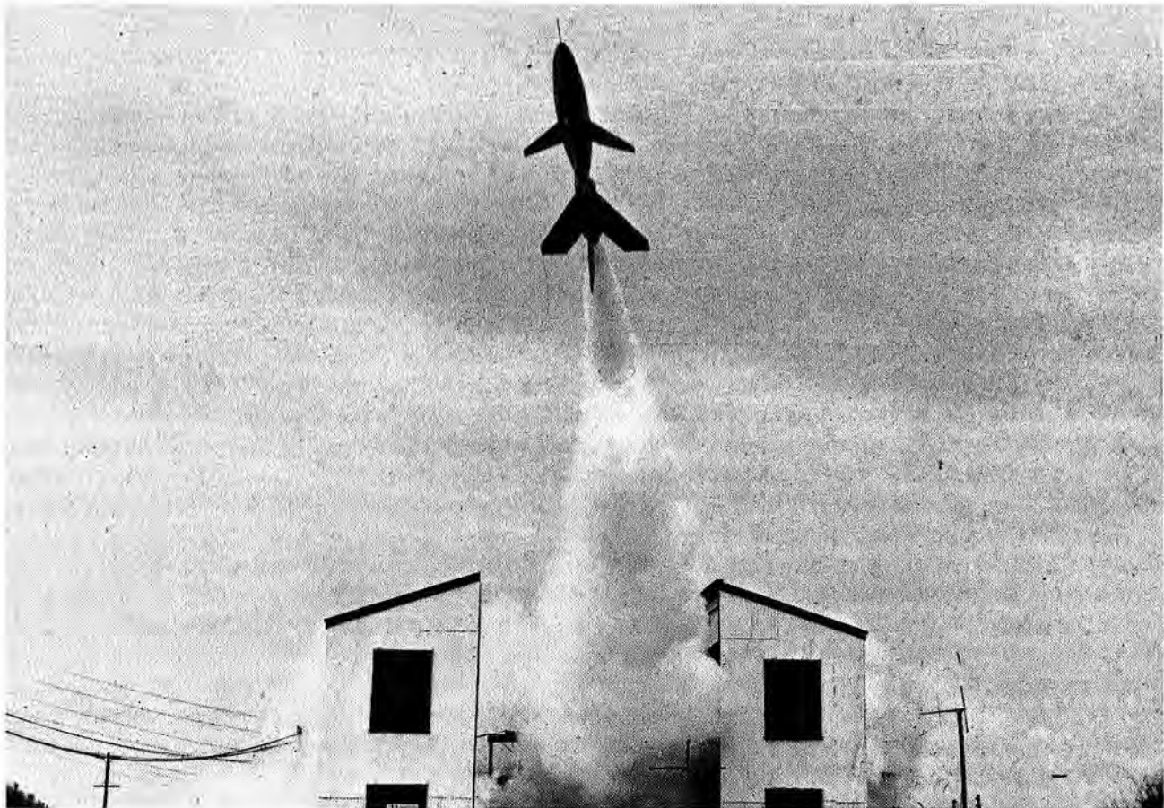
FIGURE 29. Tiamat C launching from Wallops split-house.
