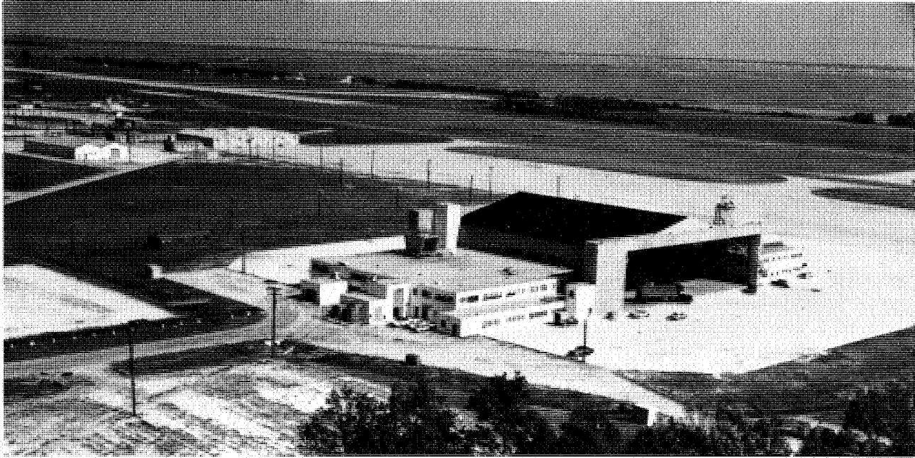
FIGURE 409. Fasron hangar (Building N-159) on Chincoteague base, converted by Wallops to range center and facility for model assembly.
